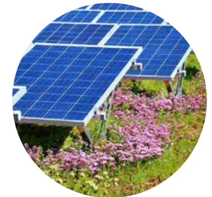
5 Green roofs with solar PV
