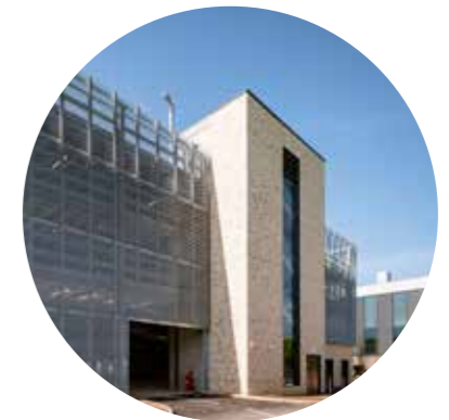
5 Multi storey carpark
